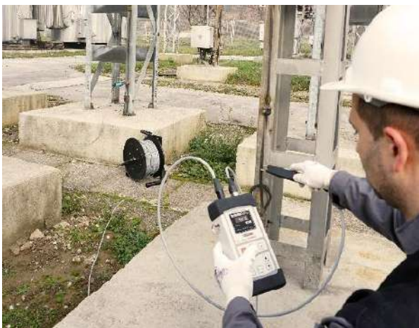
Ground grid continuity testing with RMO-EH
