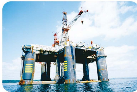
Offshore Oil Platform
