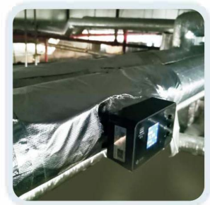
Building air conditioning flow measuring
